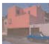
Luis Barragan , Gilardi Residence , Mexico City (Photo A.C.A)
